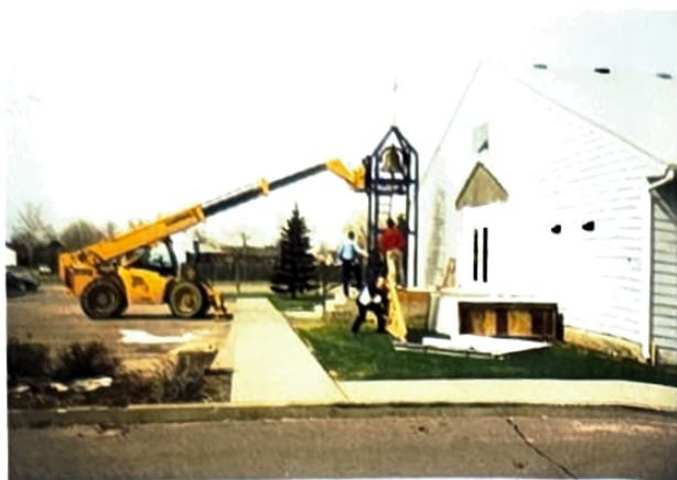
Moving the bell for the school addition- 2001
