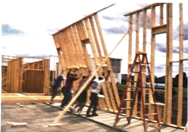
Multi-purpose Room Walls Go Up
